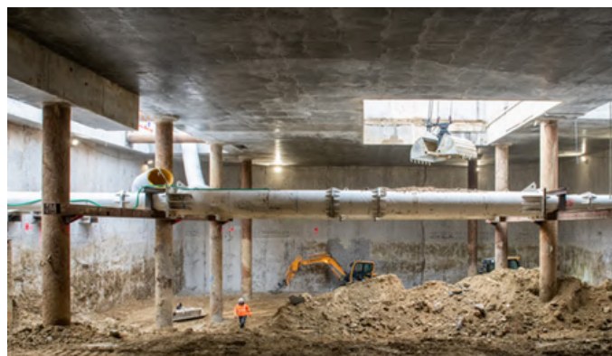
Le creusement de la station Oullins Centre, 2020
